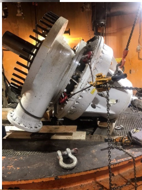
Bottom of A Digester With Outlet Device Removed
