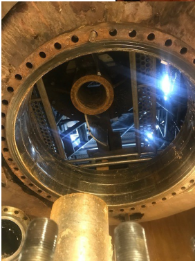
Bottom of A Digester With Outlet Device Removed
